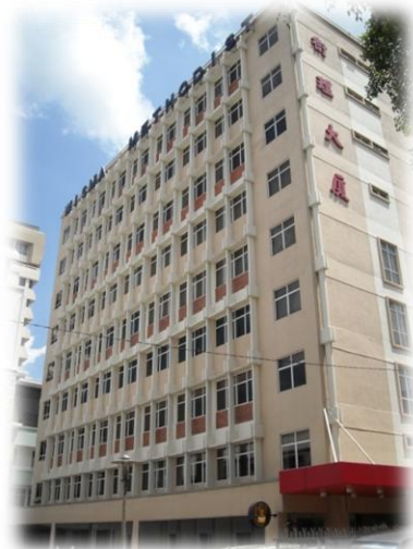
Wisma Methodist building
